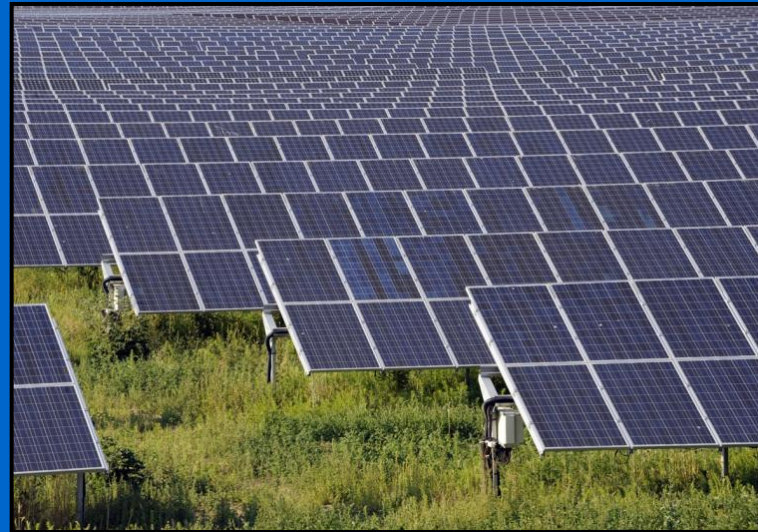
Example of rows of solar panels.
