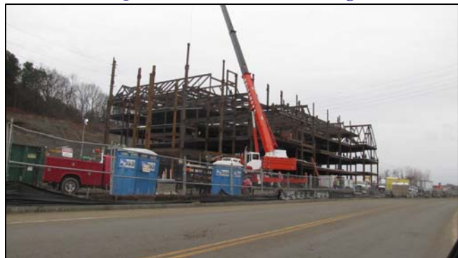
Tockwotten Home under construction, December, 2011
