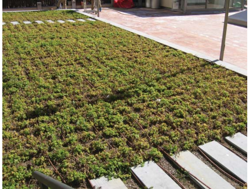
10. Green Roof, Barcelona, Spain
