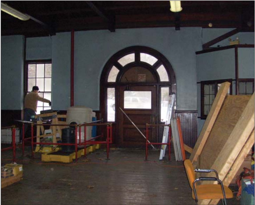
5. Pump House: Interior, Looking North
