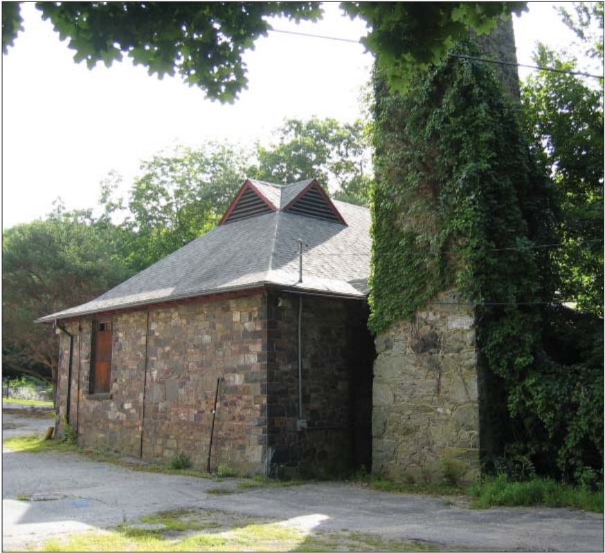
4. Pump House: Southwest Corner
