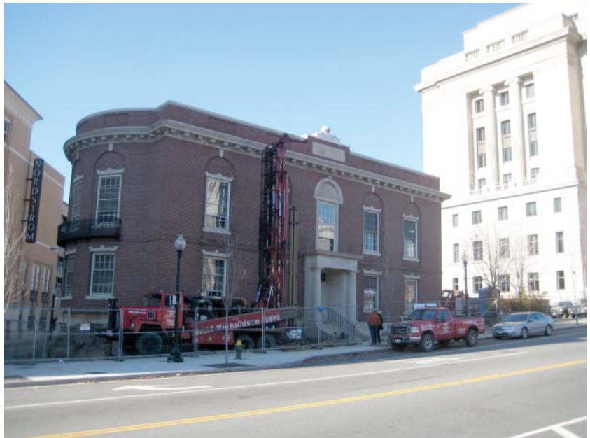
11. Geo-thermal well being dug in front of downtown Providence building
