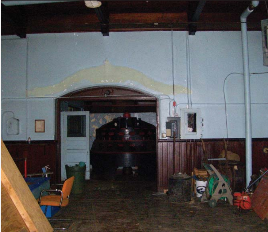
6. Pump House: Interior, Looking South
