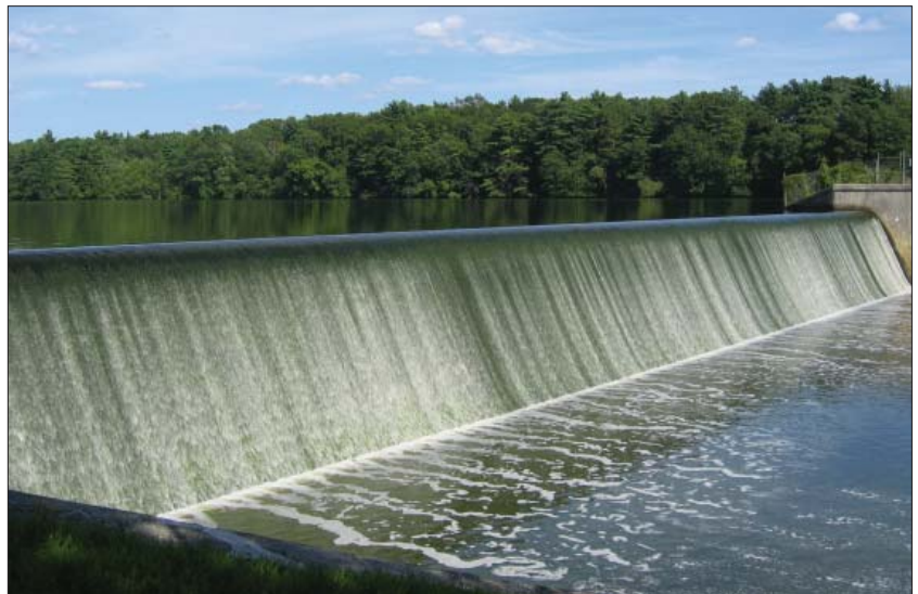
6. Turner Reservoir Dam
