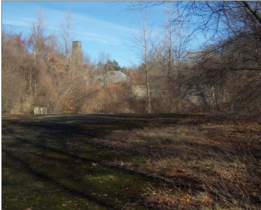
14. Top of Clearwell Tank
