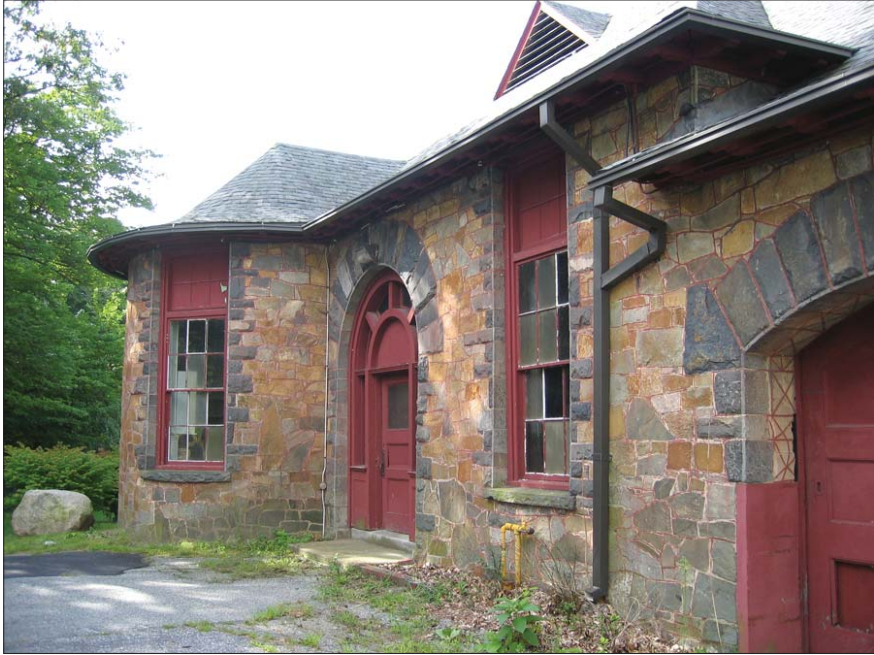
2. Pump House: Front (North) Elevation Looking East
