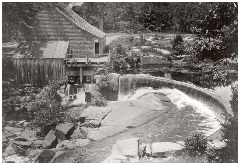
3. Historic Image of Grist Mill at Horseshoe Dam
