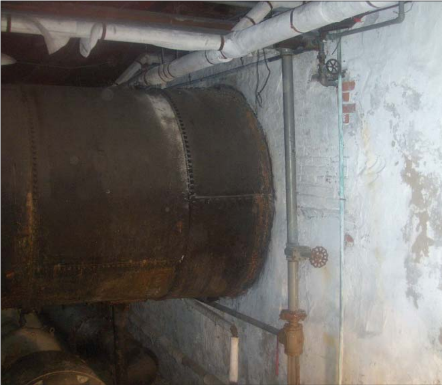
11. Pump House: Penstock Entering North Foundation Wall
