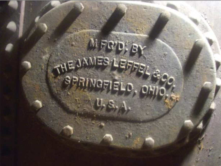
12.. Pump House: Access Cover at Leffel Turbine
