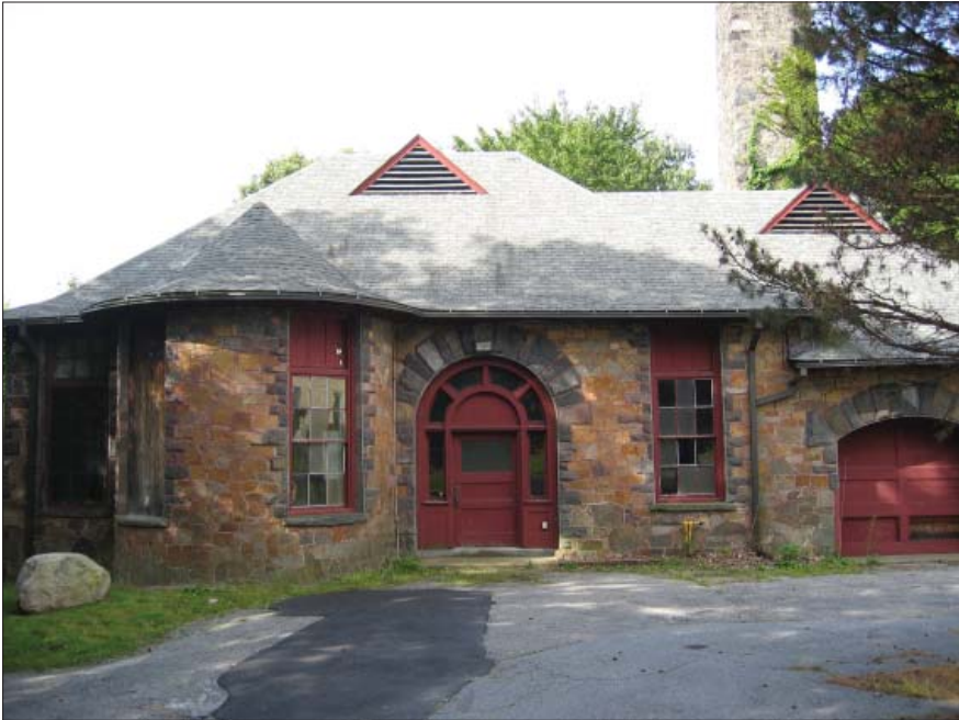
1. Pump House: Front (North) Elevation
